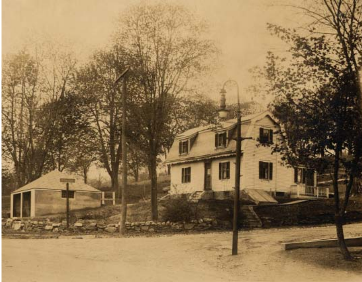
The only surviving portion of the Faneuil Estate, the Gatekeeper's House, c. 1935
