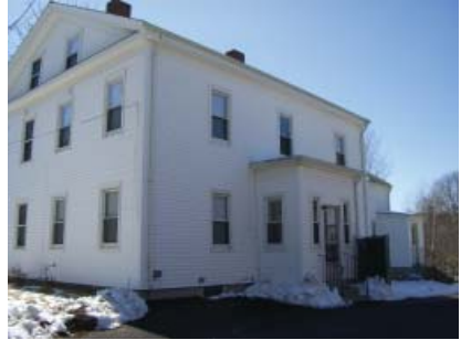
173 Foster Street, was moved across the street to this location in the 1850s. At different times the home of Hannah Foster and Fanny Fern, this building is a major Allston-Brighton literary landmark.
